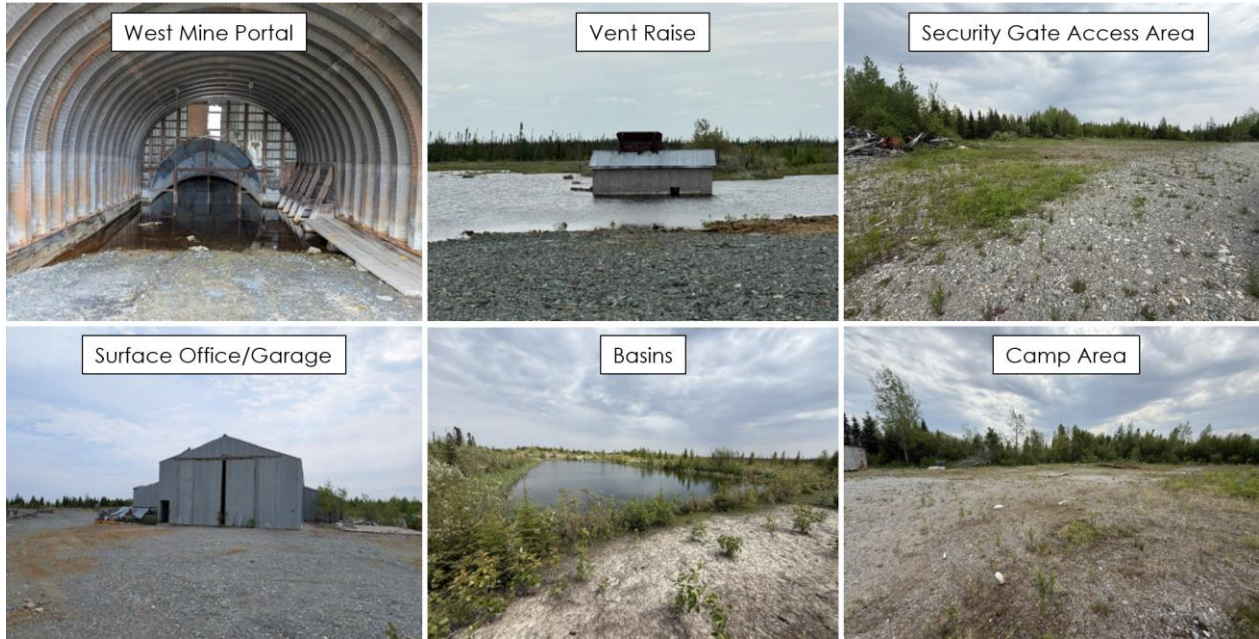
Figure 18-1: Images of existing site infrastructure, captured during site visit
